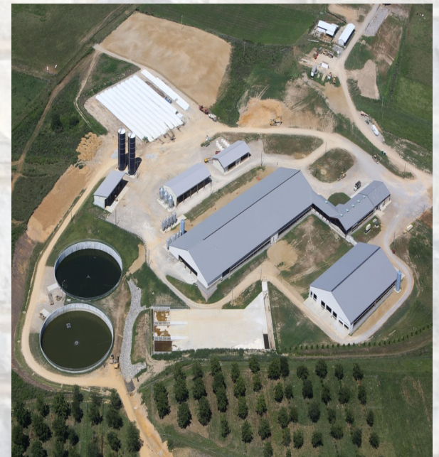
Dairy Barn Relocation - Blacksburg, VA
